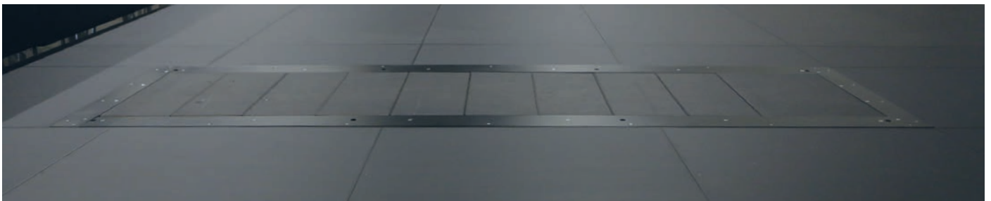
PANTOGRAPH STAIRS, FULLY INTEGRATED IN THE STAGE FLOOR
